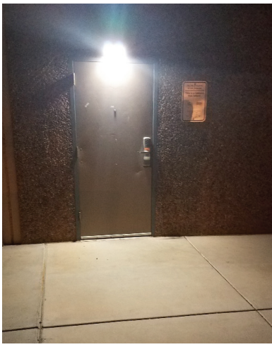
SOLAR WALL PACK - 7W, 700 LUMENS
