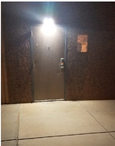
SOLAR WALL PACK - 7W, 700 LUMENS
